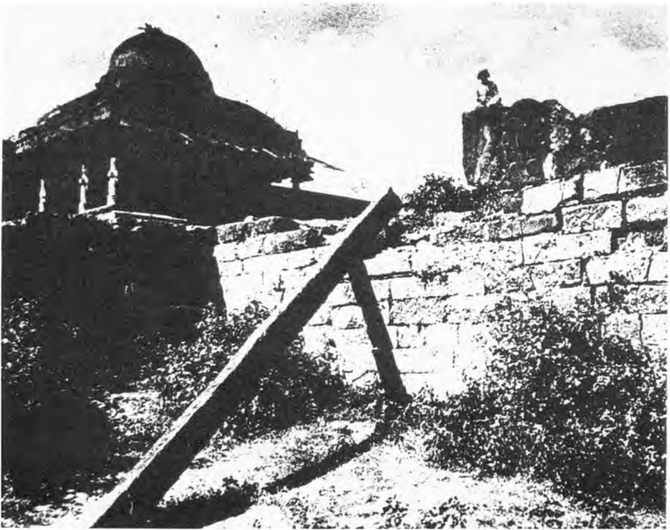
Fig. 2: Photograph taken in the early 1900s showing the longest piece of the Dhar iron pillar lying in a sloping position against the masonry terrace in front of the Lāṭ Masjid. This piece remained in this position from 1531 AD till about 1980 AD. Photograph courtesy: Archaeological Survey of India.
