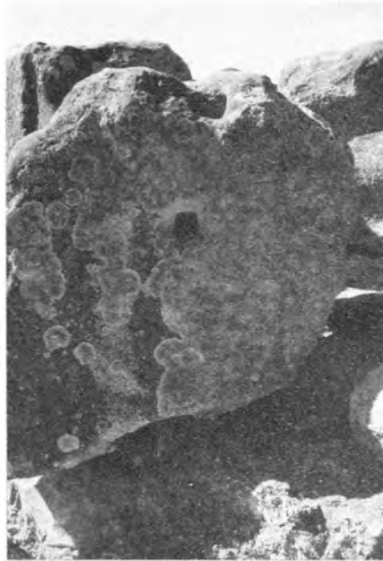
Fig. 14: Hollow cylindrical slot provided at the bottom of one of the stone boulders that were originally used for holding erect the Dhar iron pillar. This hollow slot was used also for gripping the stone boulder to the masonry basement by means of an insert, similar to the pillar clamped with an insert to the stone boulders.
